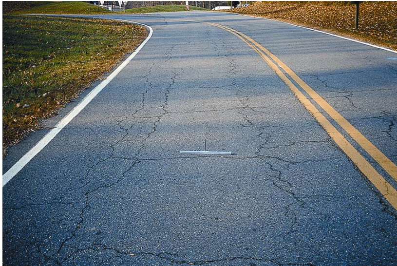
Figure 7 - Block Cracking
