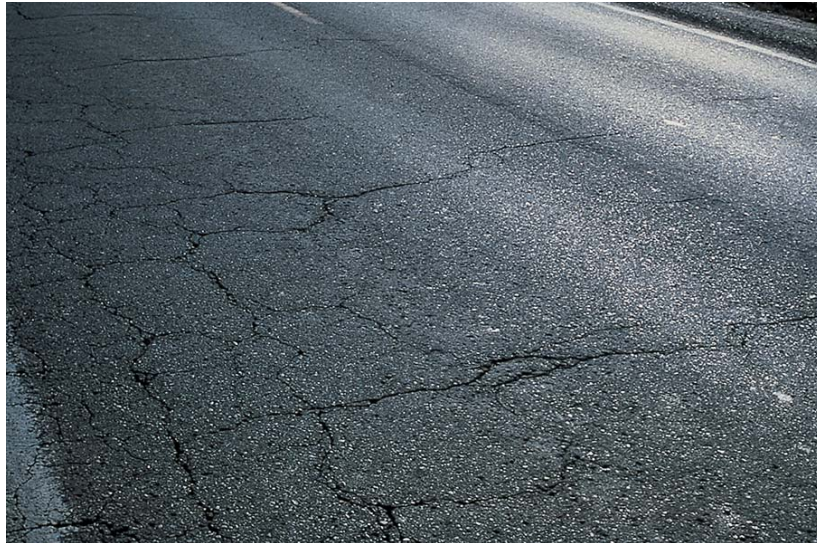
Figure 8 - Block Cracking
