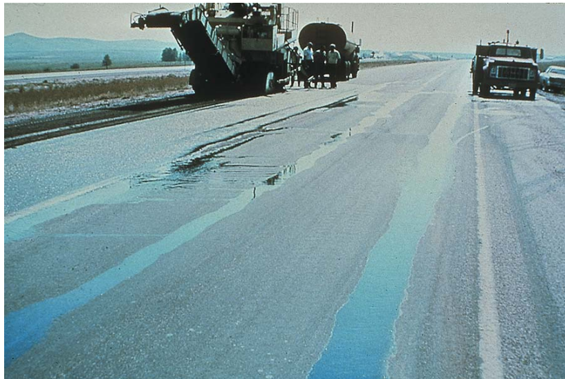
Figure 22 - Standing Water in Ruts
