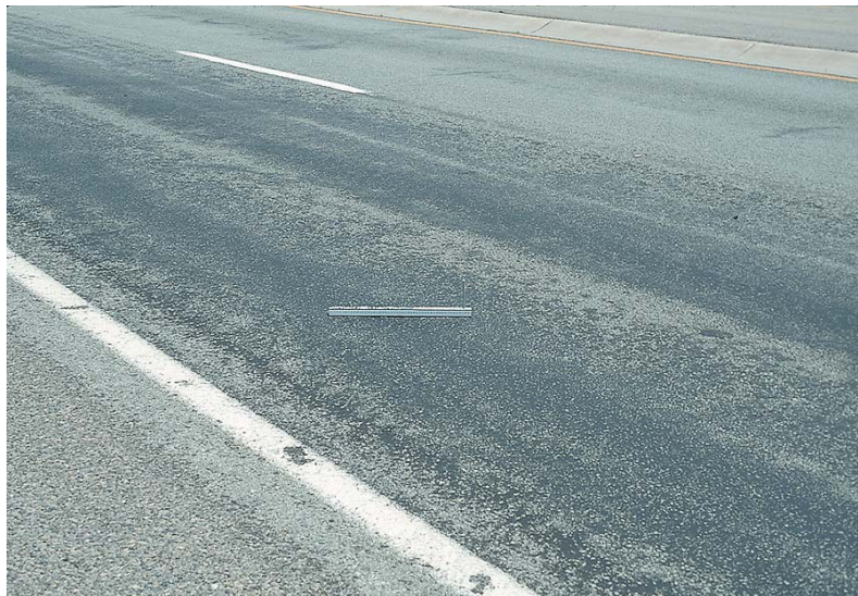
Figure 26 - Loss of Texture
