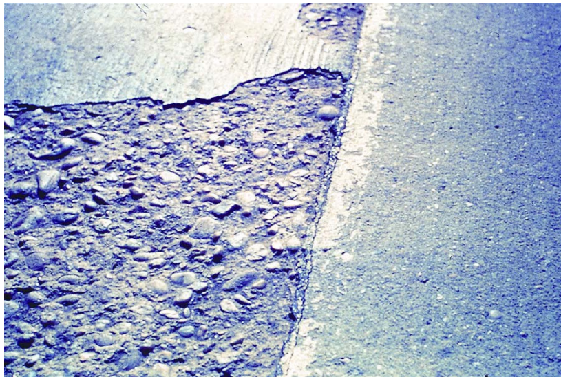
Figure 53 – Scaling
