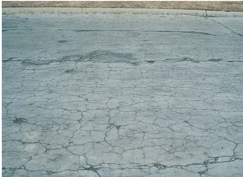
Figure 52 - Map Cracking
